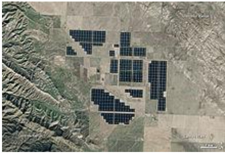
Figure 4 Satellite image of the 550-megawatt Topaz Solar Farm in California, USA
