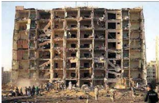
Fig.1 Building collasps in Khobar Towers due to blast action (1996)
