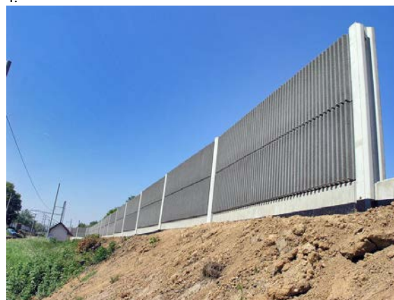
Fig. 4: Absorption wall with the surface of the autoclaved cellullar concrete (porous concrete) (Fotogalerie / Liadur.cz, 2012)
