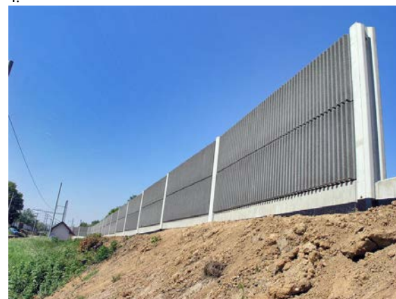
Fig. 4: Absorption wall with the surface of the autoclaved cellular concrete (porous concrete) (Fotogalerie | Liadur.cz, 2012)
