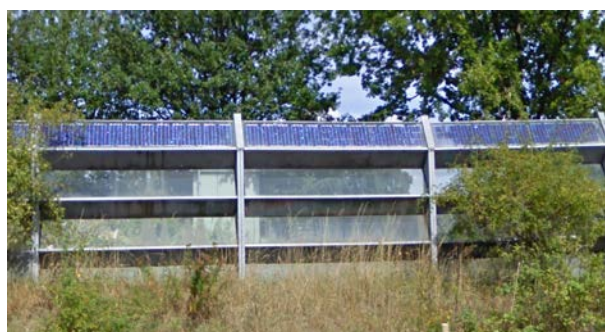
Fig. 6: A combination of reflective and absorptive barrier in Copenhagen, Denmark
