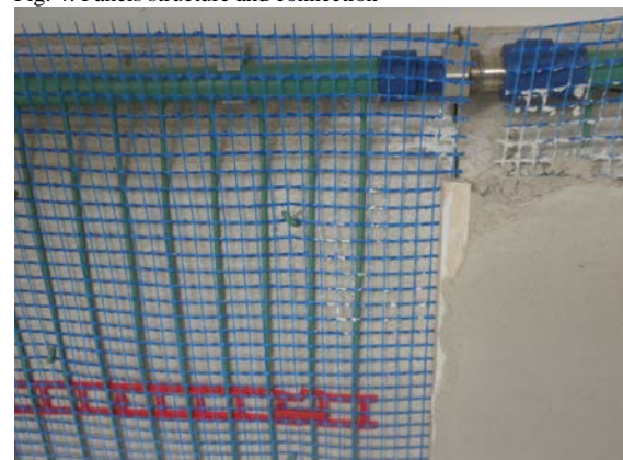
Fig. 4: Panels structure and connection
