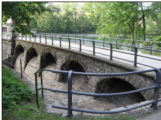
Fig.2. Safety spillway and chute
