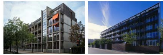
Figure 1. Germany. Reconstructed large-block residential buildings [10]
