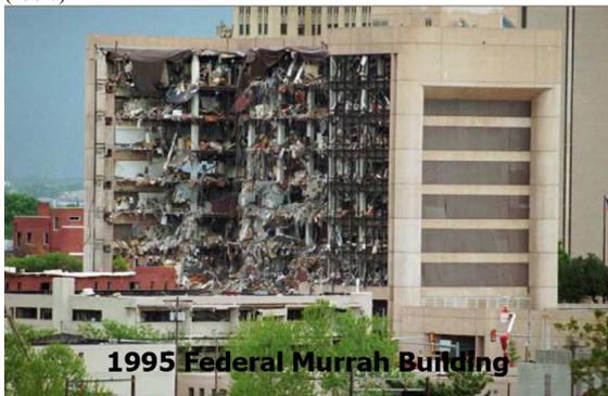
Fig.2 Building of Federal Murrah Building after blast attack (1996)
