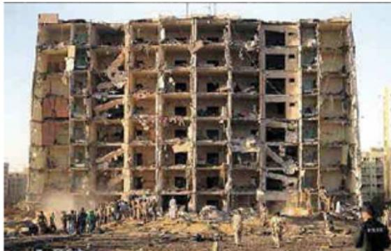
Fig.1 Building collaps in Khobar Towers due to blast action (1996)
