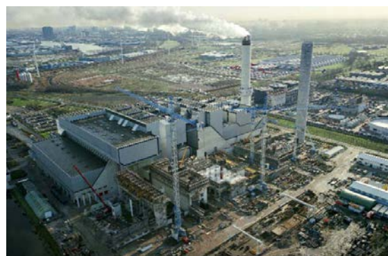
Fig. 3. Waste incineration plant, Amsterdam, Netherlands, source: ECOFYS
