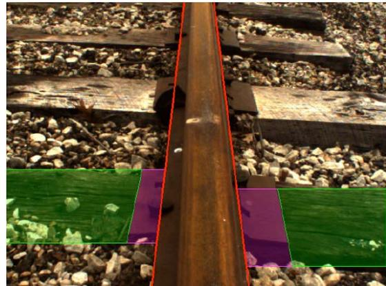
Figure 2: Delineated Tie and Tie Plate location Estimations
