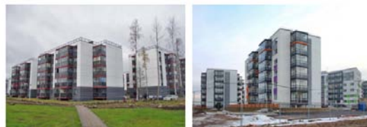
Figure 2. Finland. Residential area of reconstructed large-panel buildings [10]
